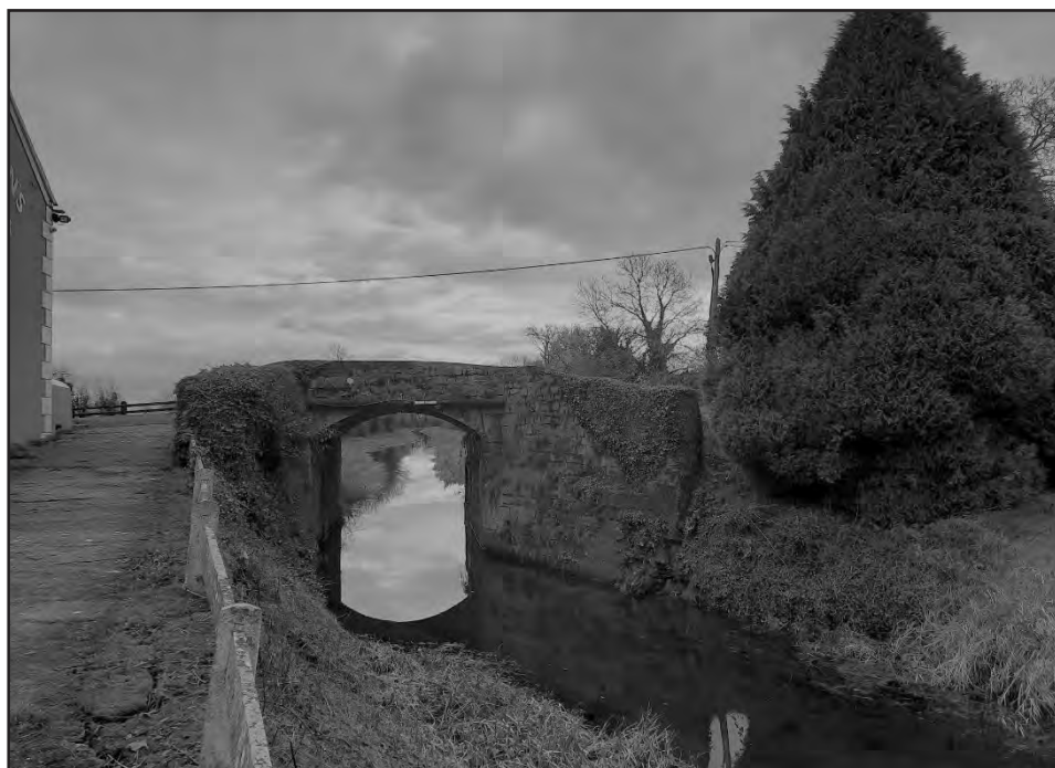
Milltown Canal Bridge
